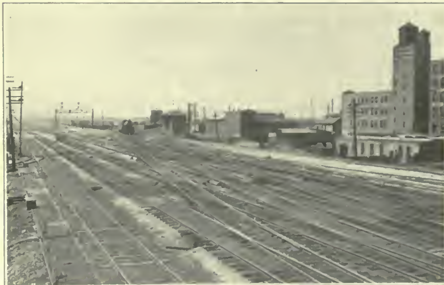
FIG. 262. GRADE CROSSINGS. Crossing of the Chicago & North Western Railway and the Chicago, Milwaukee & St. Paul Railway, at Western Avenue.
